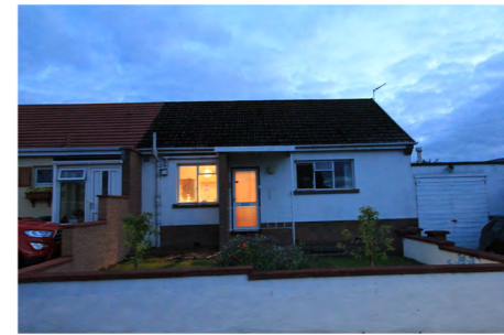
House on Cramond Crescent in need of gable
